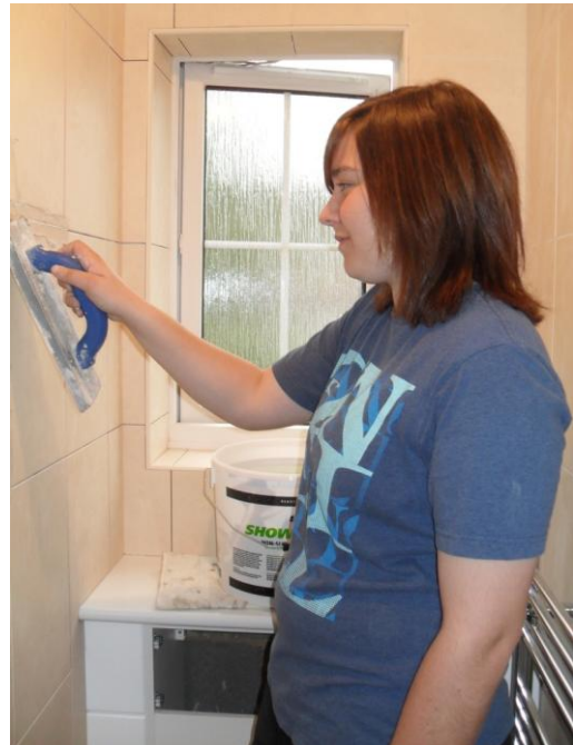
Megan doing grout work
